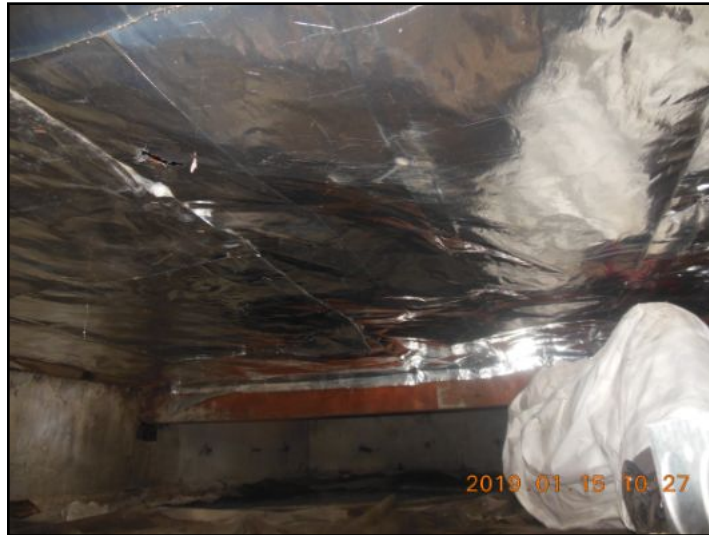
Subflooring invisible due to finishing with aluminum foil covering
