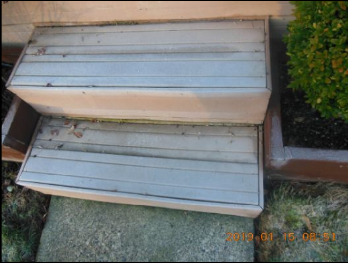
Stairs of front patio
