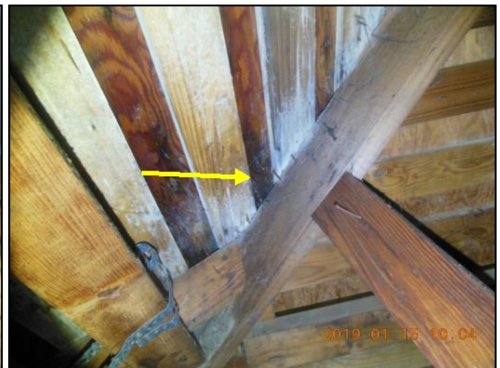
Potential biogrowth/mold
