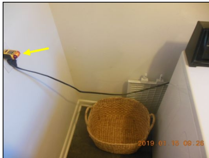
Outlet for washer has open ground
