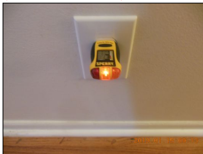
Outlets with open ground
